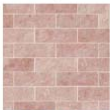
Architectural masonry in pink tone to the lower ground floor areas
