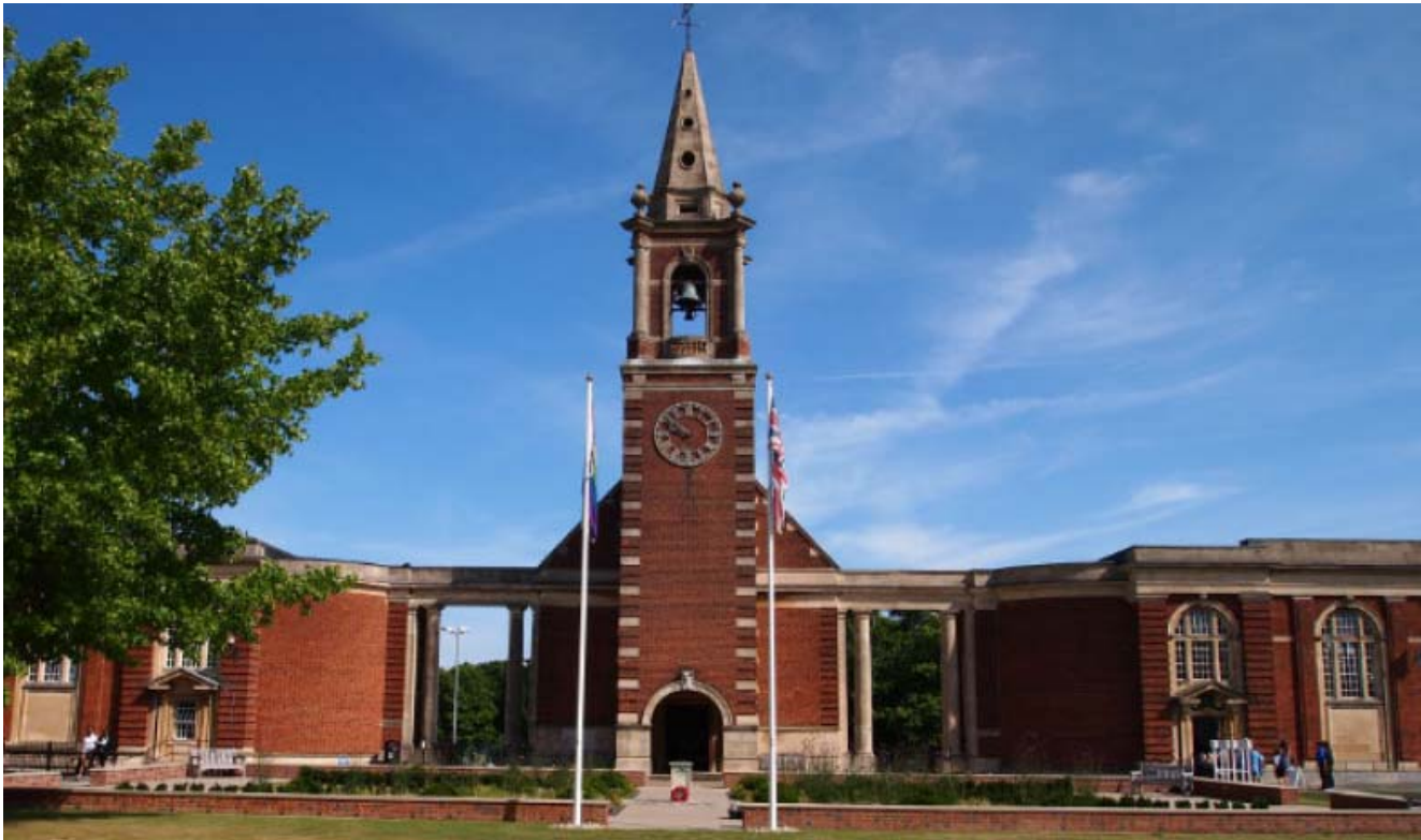
Figure 12: Rounded features to Chapel, with Great Hall to the left and Dining Hall to the right
